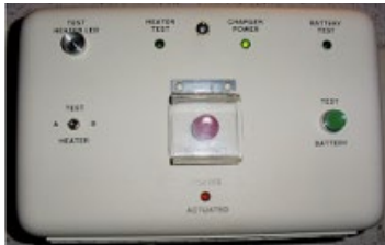
Figure 27. (a) Universal symbol used for emergency table stop safety switch. (b) Example of an emergency power off safety switch. (c-d) Examples of Quench (emergency field run-down) units (Source: GE and Siemens Operator Manuals)
