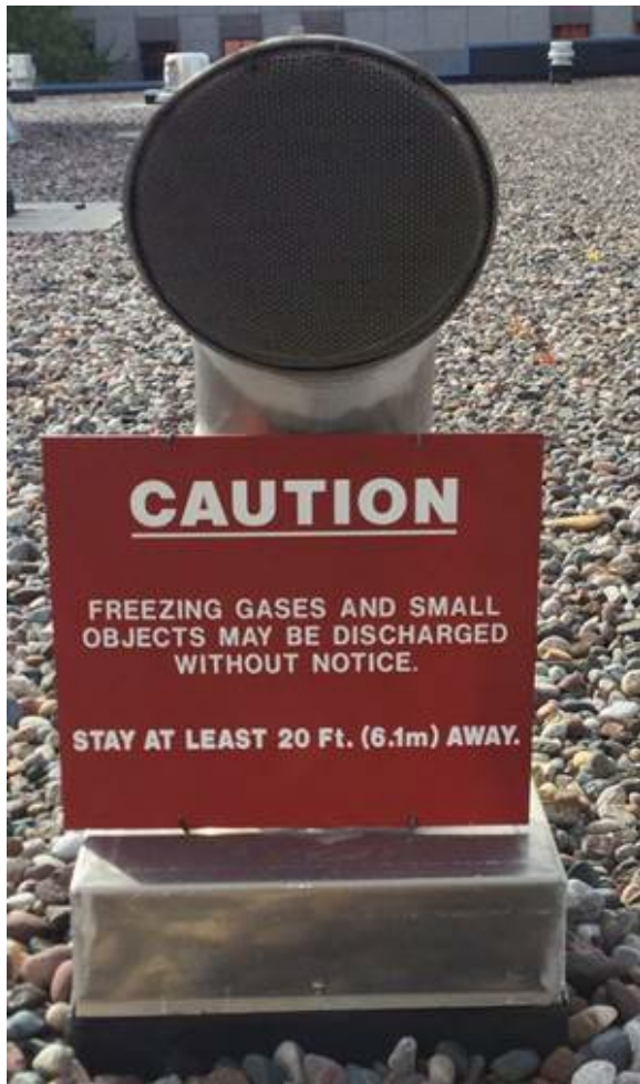
Figure 4: Example of cryogen vent labeling.
