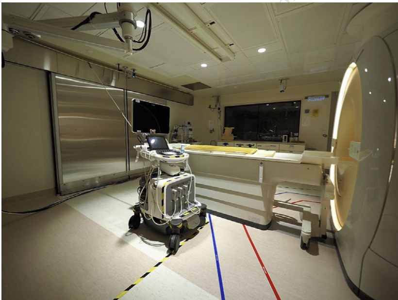
1807 1808 Figure 19. Tethering and placement of anesthesia equipment in Zone IV. Red arrow points to the tether. Black arrow 1809 represents the 200-gauss line.
